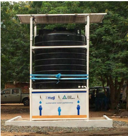
The solar-powered mechanized borehole
